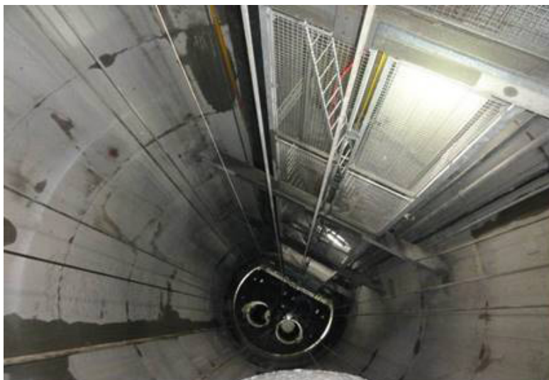
Slika / Figure 4, Okno, skela / Shaft, ladder compartment
