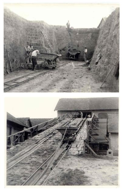
Kanjiža, up - works on excavation and loading of clay, down - brick drive slipway
